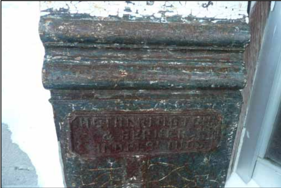
101 S. Main Street, Cast iron pilaster detail
